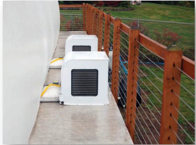
Dual Commercial Ameri-Dome Heating System
