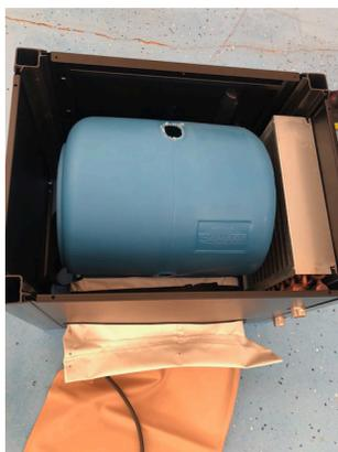
11. Pull the white boot flange completely through the opening and reattach it to the Dome heater using the same screw holes that originally were removed.
