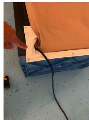
12. This picture shows how the power cord should be routed through the boot (there will also be a clear pressure sensor tube on residential domes).
