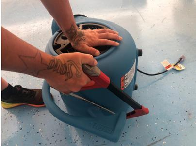
1. Use a hacksaw to completely remove the handle of the blower. Cut it off flush with the body of the blower (this will not affect the blower performance or its longevity).
