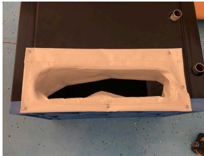
5. Remove the white vinyl boot from the heater housing by removing the attachment screws.
